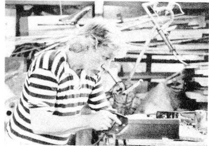
The Old Bakehouse Trust, Oxford: a carpenter and an electrician (overleaf) at work in the workshops
